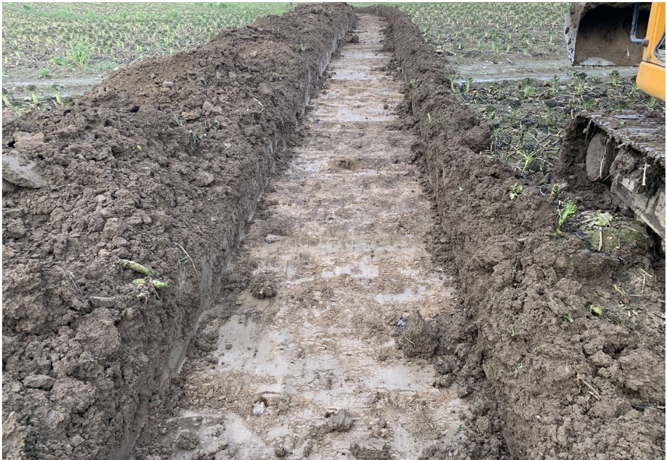
Plate 41: Area 1C: Test Trench 33 facing north
