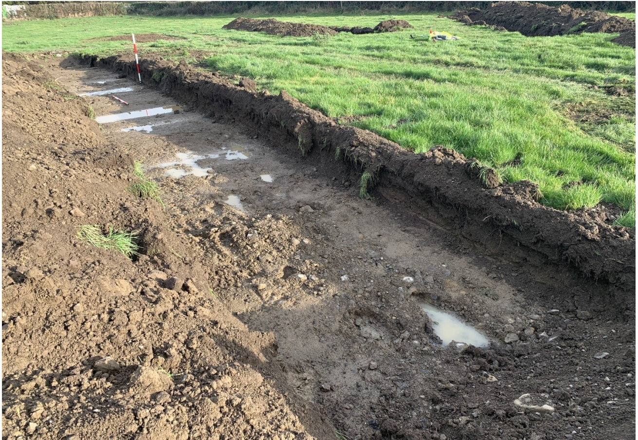
Plate 15: Area 1A: Test Trench 12 facing north-east
