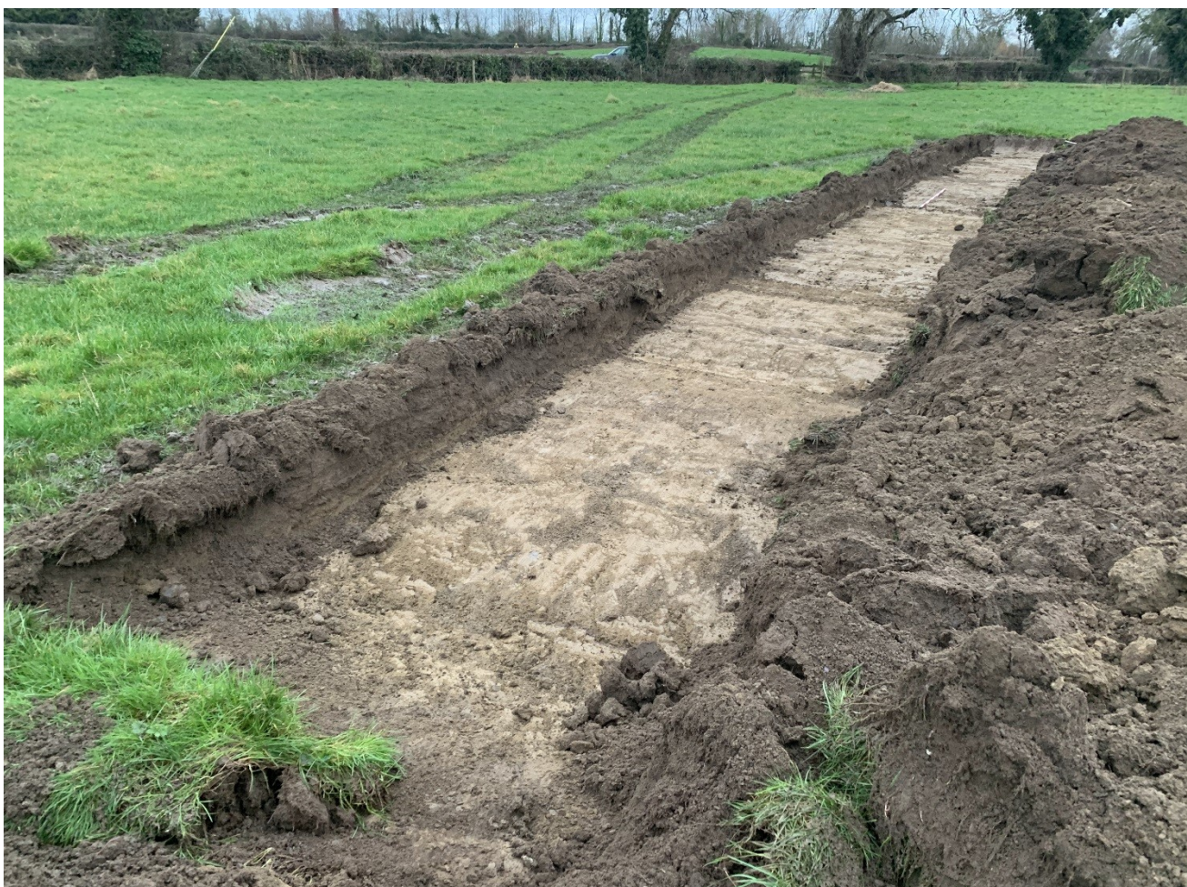
Plate 24: Area 1A: Test Trench 24, facing southeast
