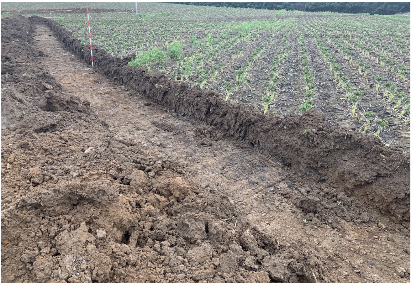
Plate 46: Area 1C: Test Trench 37 facing north-west
