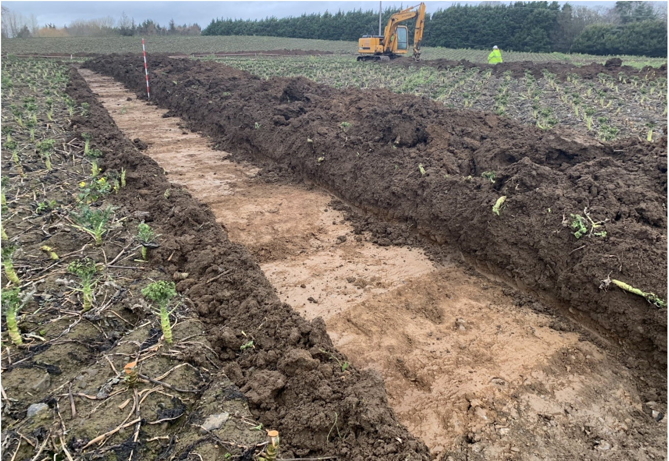
Plate 45: Area 1C: Test Trench 36 facing north-west
